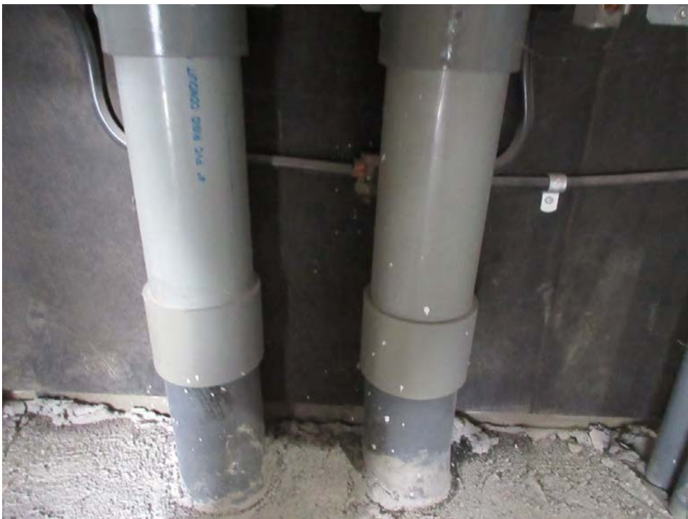
11. View of Service Conductors/Raceways
