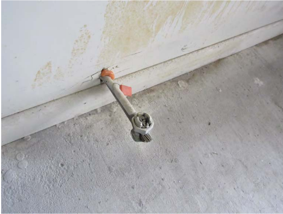
9. View of Grounding of Service
